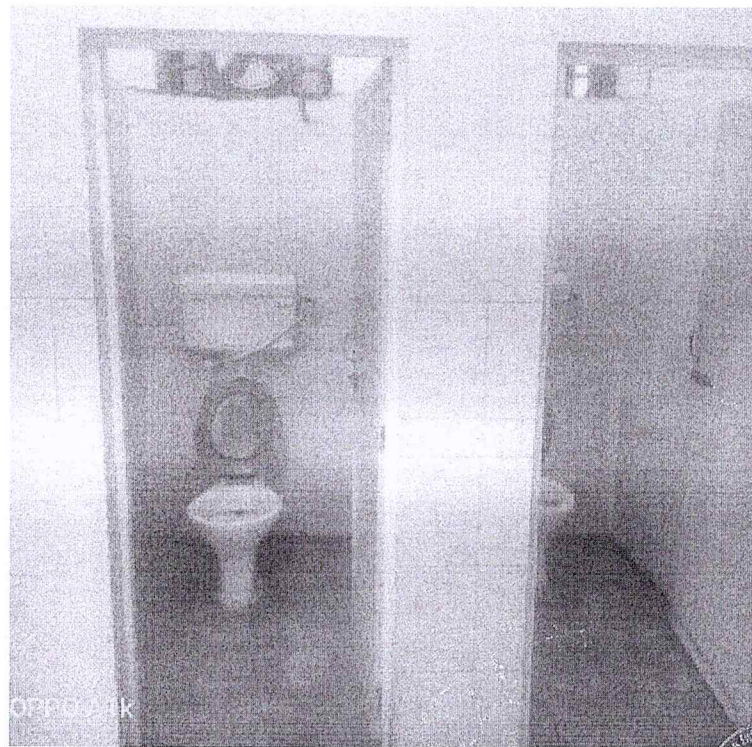
Site photograph 3 Campus Toilets
